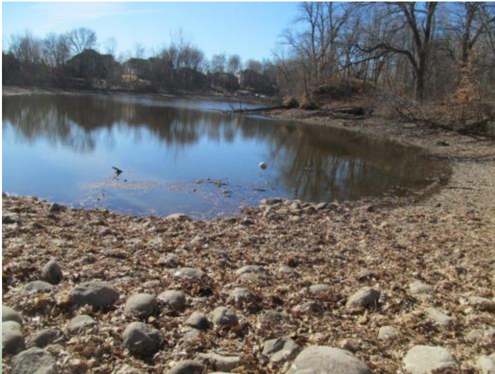
Lake side of dam 2 weeks after close
