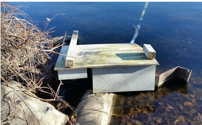
Present condition of the power meter panel after yanked into the lake on November 28 th .
